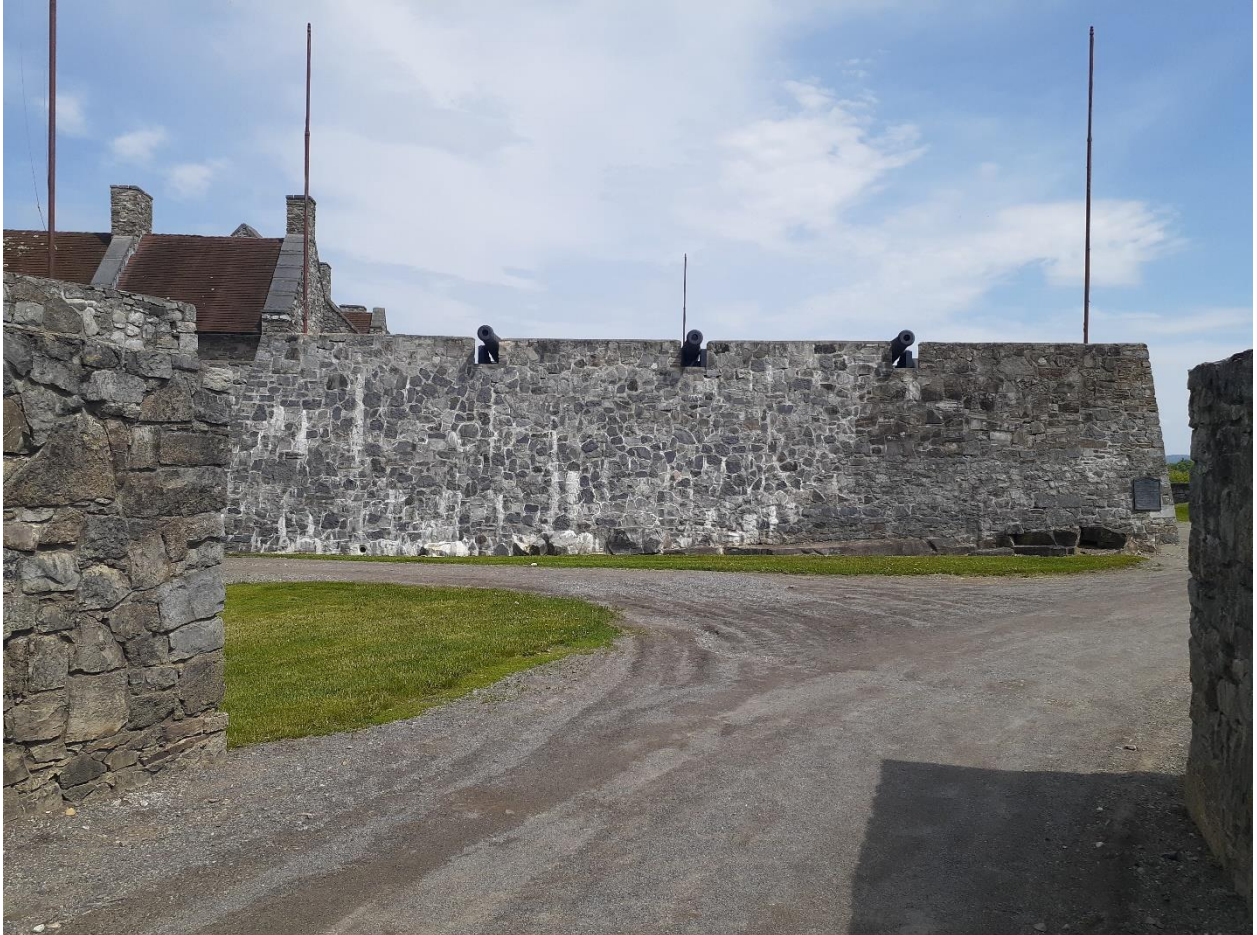
Figure 2 View from the main entrance to the site which emphasizes the works done in the style of Vauban.
